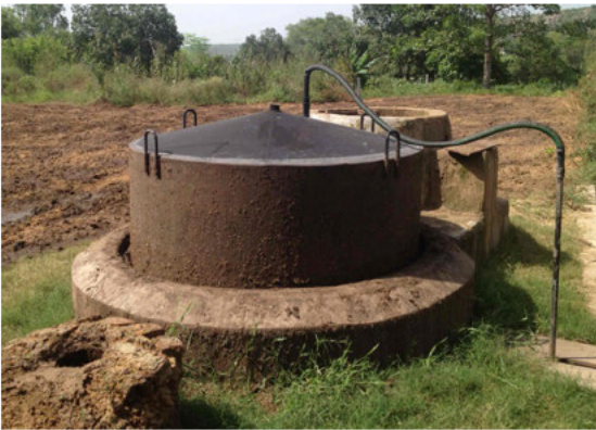
A gobar gas storage drum
